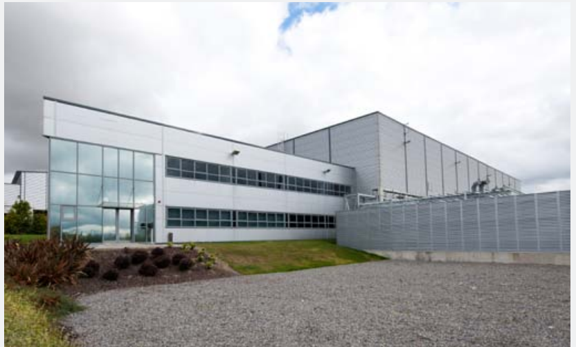
Image Exterior of Data Centre
